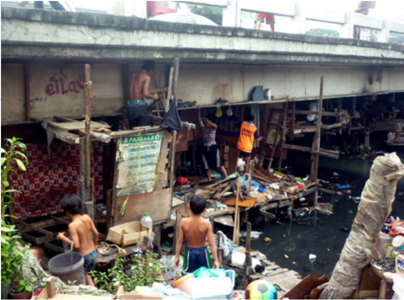
2014: Homes under the bridge of the Tulay community being dismantled.
