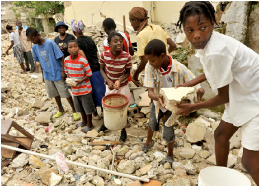
After the earthquake, everyone worked together to clear the rubble.
