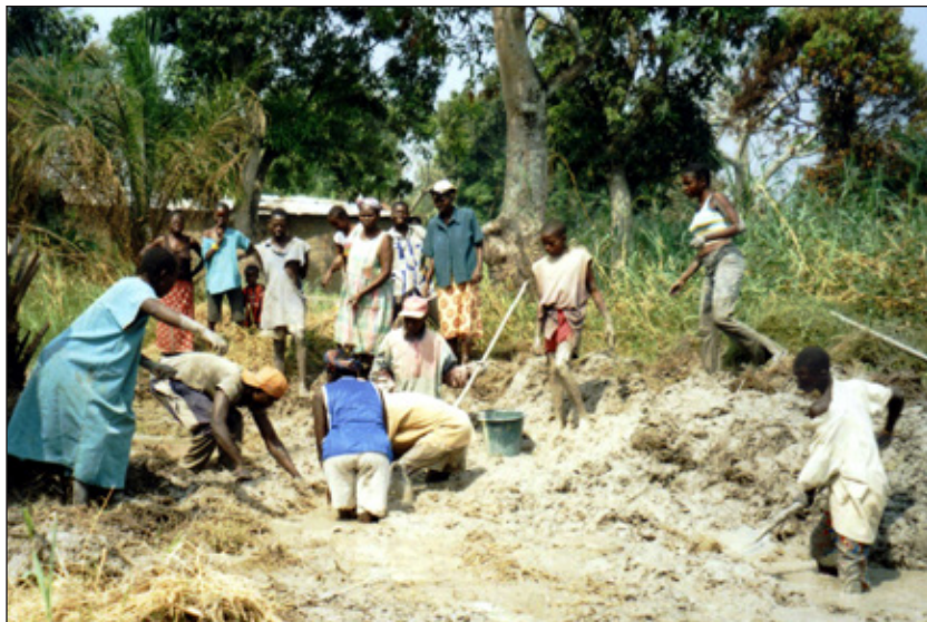
In 2007, our members launched a community project to clear drainage ditches.
