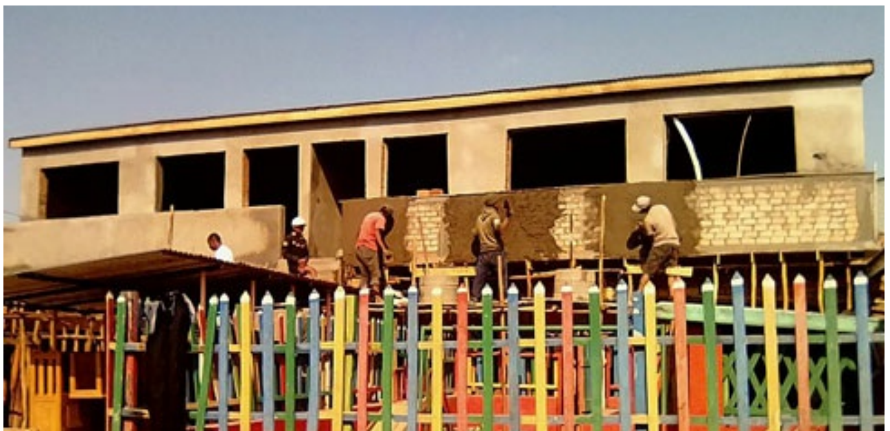
School project under construction.
